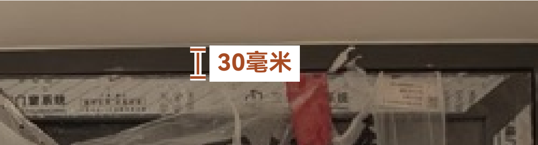
纱窗顶部缝隙放大
